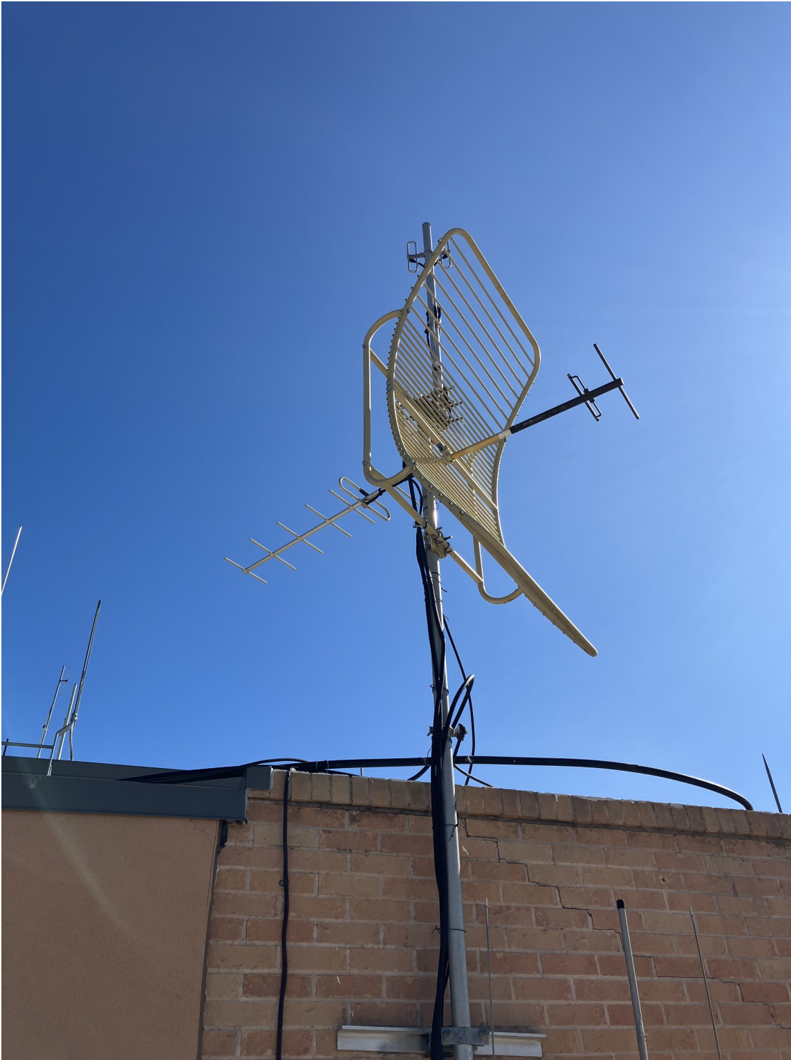
Figure 1: Multi-user antenna farm: DB-408 at top Commercial repeater; SRL 307 Yagi and Scala PR-410 Paraflector Ham Radio Links. Site is on a locked roof top: Controlled Access.
